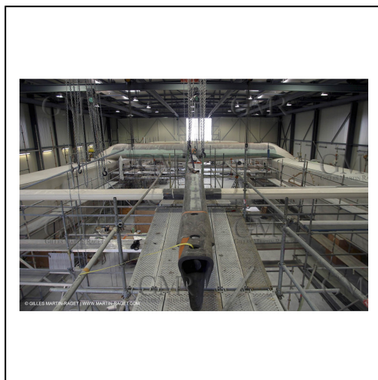
Vannes - Chantier Multiplast - Construction Orange II *** Vannes - Multiplast Boatyard - Orange II construction
