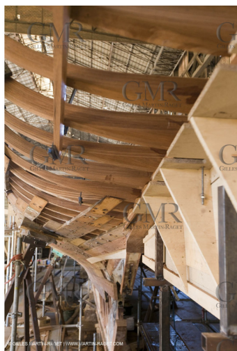
14/12/2007 - La Ciotat (FRA, 13) - Restauration de Mariska aux "Charpentiers réunis"***14/12/2007 - La Ciotat (FRA, 13) - Mariska refit at "Charpentiers Réunis" boatyard
